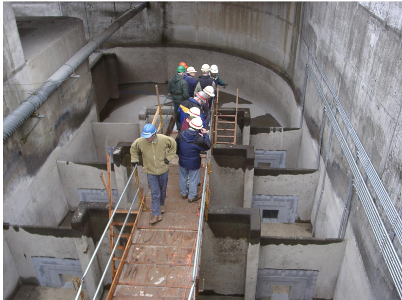
Installing adult detectors in the Washington shore ladder at Bonneville Dam
